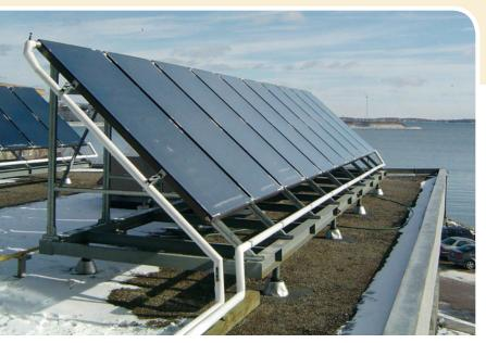
Solar thermal panels allow RainTree's ESTES to capture energy directly from the sun.
