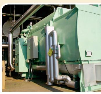
ESTES uses adsorption chillers to cool indoor space at greatly reduced cost.
